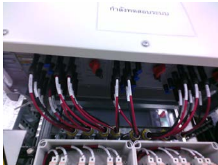
Scan the heat of MC4 Under the inverter.
